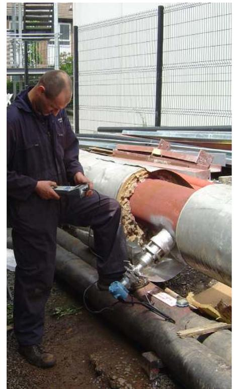
*Newly installed Rosemount 3095MFA averaging pitot tube steam flow meter being commissioned*
