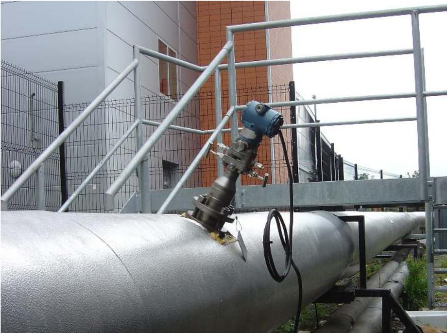
*Rosemount 3095MFA steam meter providing stable and accurate flow readings, even at low flow velocities*
